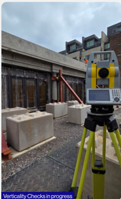
Verticality Checks in progress
