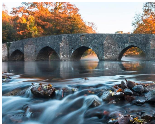
New Bridge, Merthyr Mawr, Bridgend
