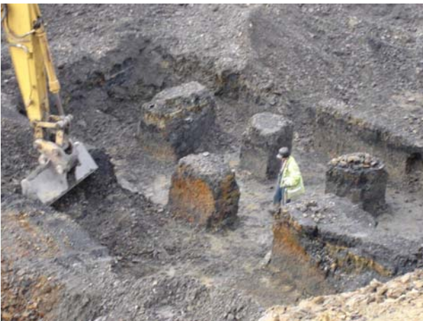
Pillars of coal being extracted as part of ground works: prevents sterilisation and effective method of remediating unstable ground caused by former coal workings
