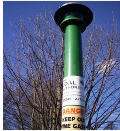
Mine Gas Vents
