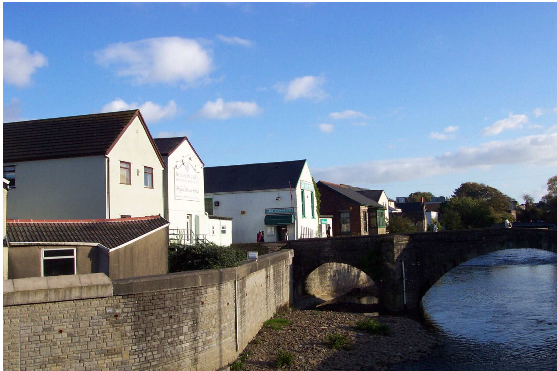
Rear of Dunraven Place Properties
