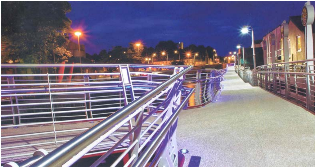
River Ogmore Walkway and Bridge
