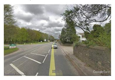
${\it Image 19-Tactile paving and dropped kerbs absent from eastern access. Footway on eastern side is substandard (too narrow) (© Google Streetview 05/18)}$
