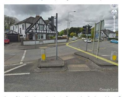
Image 21 – No advanced cycle stop lines at signalised roundabout. Dropper kerbs, tactile paving and refuge island crossings on southern, western and northern arms. Puffin crossing incorporated into signals on eastern arm. (© Google Streetview 05/18)
