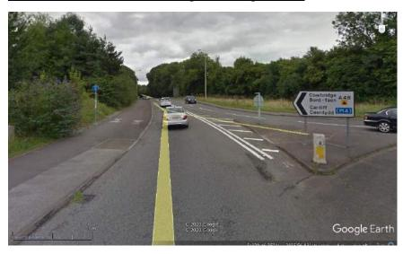
Image 1 – Shared Cycle Path, dropped kerbs and tactile paving crossings at Broadlands Roundabout facing east along A48 (© Google Streetview 08/16)
