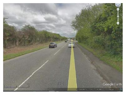
Image 25 – Missing footway on northern side of A48 and sections of narrowed footways on southern side of A48 between Hernston Lane and Picton Roundabout (© Google Streetview 05/18)
