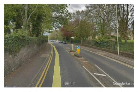
Image 13 – Pedestrian crossing with tactile paving, dropped kerbs and refuge island. (© Google Streetview 05/18)
