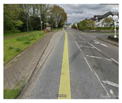
Image 20 — Tactile paving absent from Priory Avenue junction. Footway of an acceptable width commences on western side of Ewenny Road (© Google Streetview 05/18)
