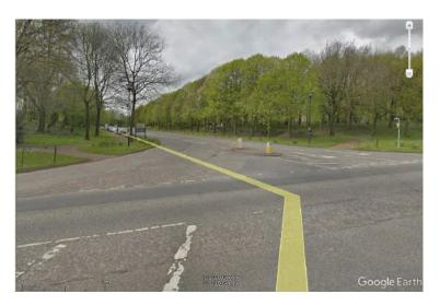
Image 18 – Dropped kerbs and pedestrian refuge island at Technology Drive. Tactile paving absent. (© Google Streetview 05/18)
