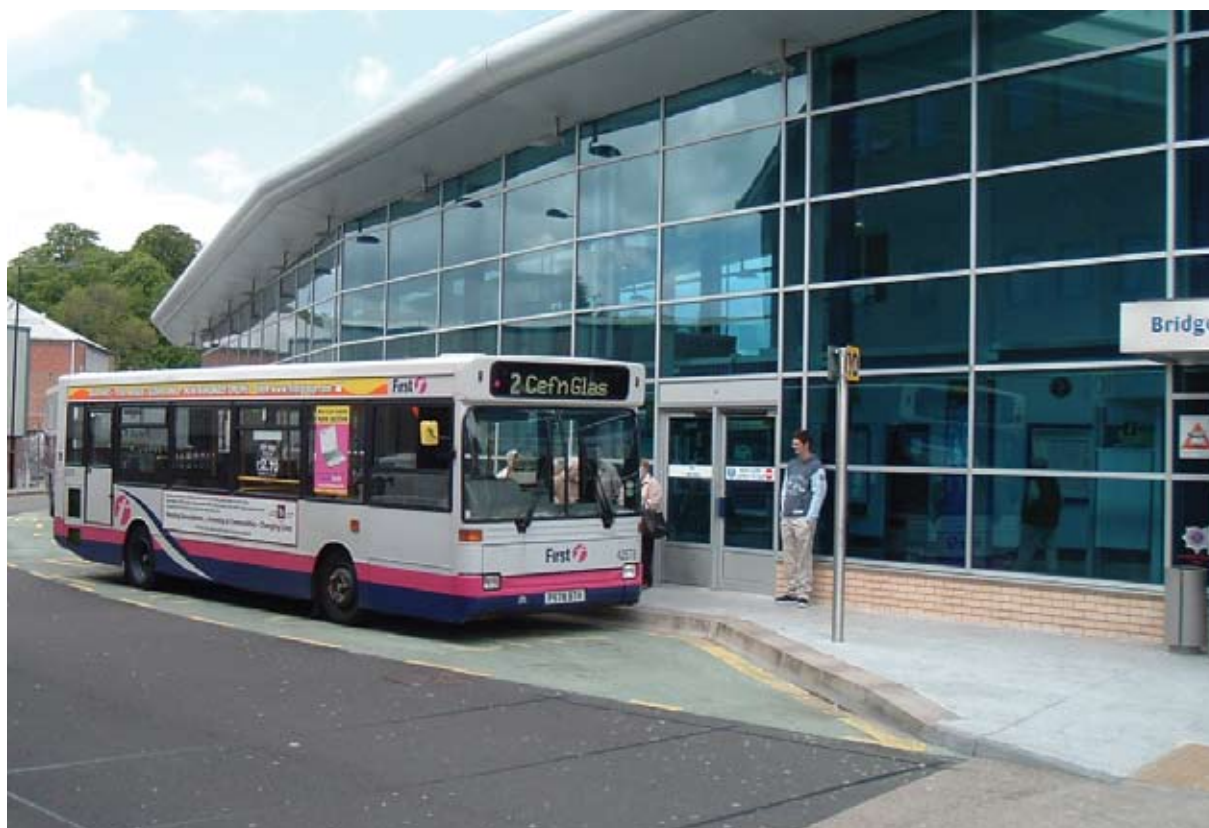
Bridgend Bus Station
