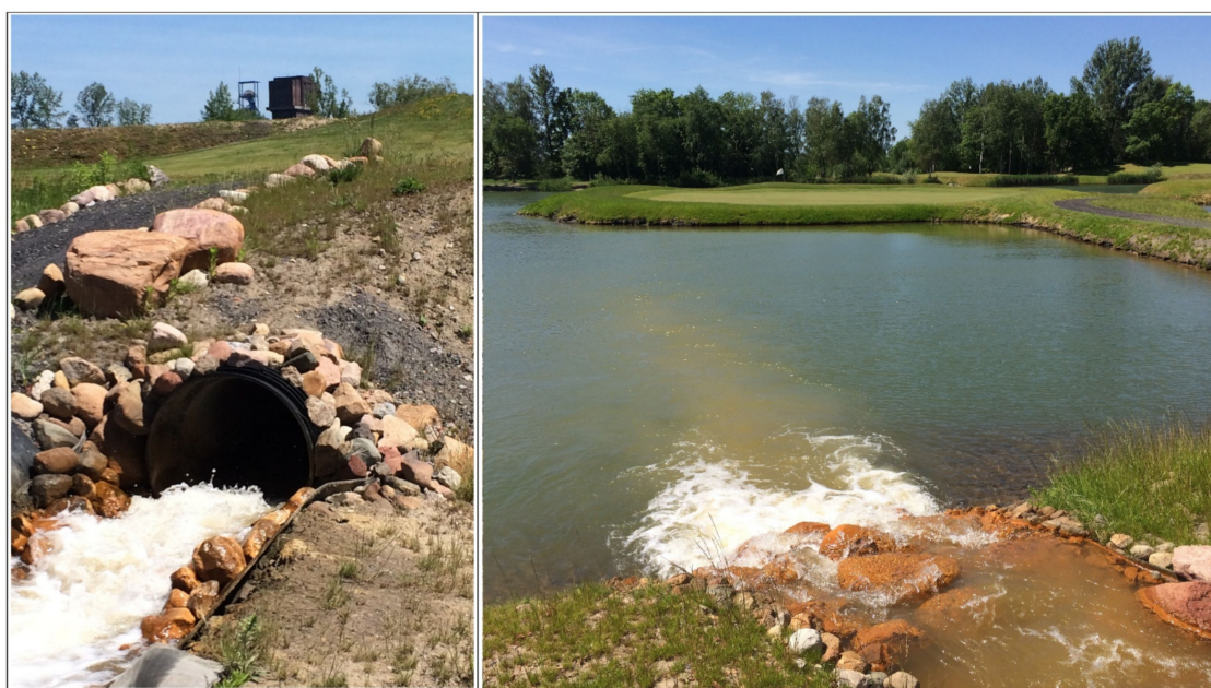
Figure 6. The pumped mine water discharge from Ewa shaft in Bytom, Poland (left), and its outfall into a lake within the ARMADA housing development complex (right). Reprinted with permission from ref. [70]. Copyright 2017 David Banks.
