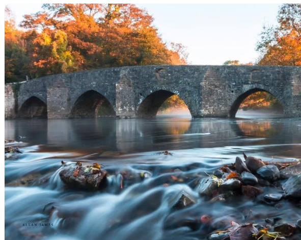
New Bridge, Merthyr Mawr, Bridgend
