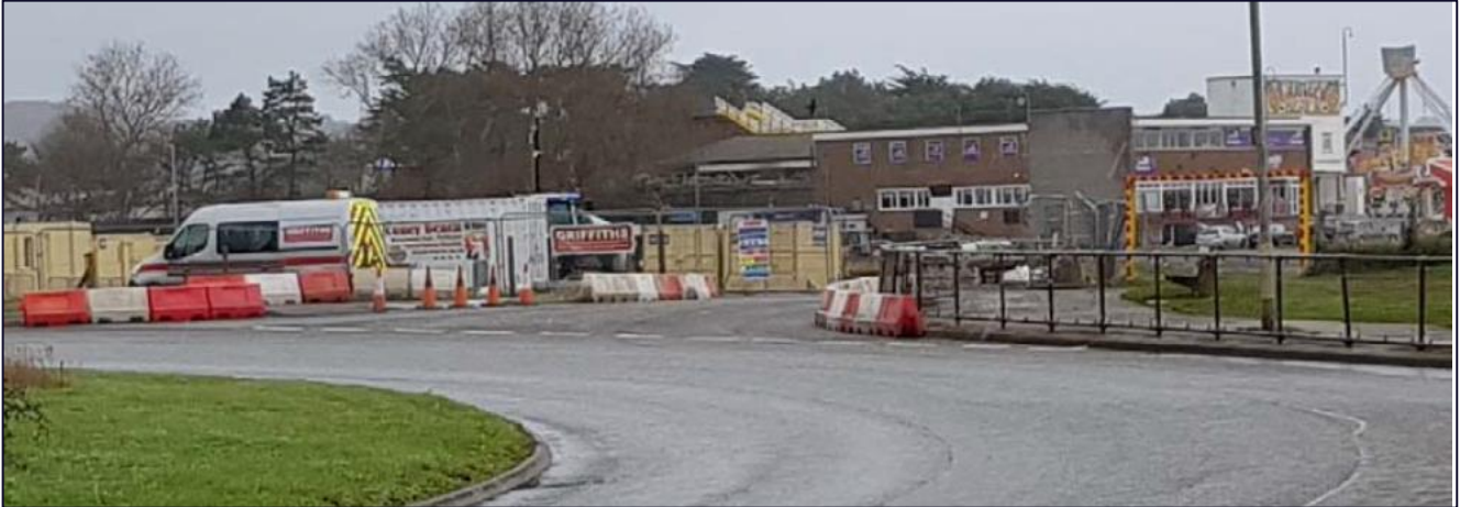
Photo 21 – Existing Access of the A4016 Roundabout
