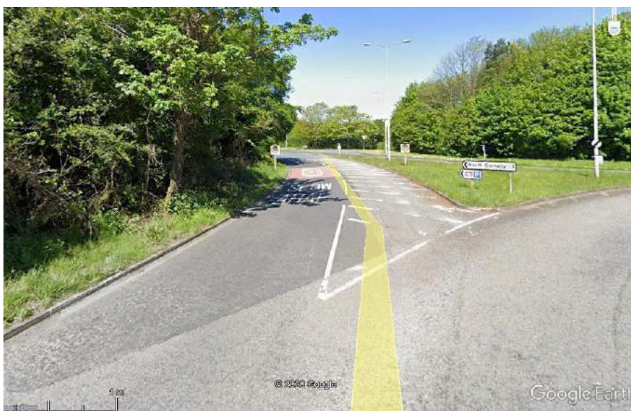
Image 2 – Lack of footway provision from roundabout towards North Cornelly (© Google Streetview 05/18)
