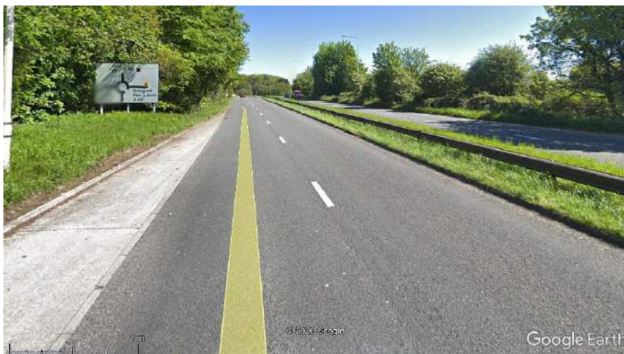
Image 1 – Lack of footway provision or crossings on A4229 (© Google Streetview 05/18)
