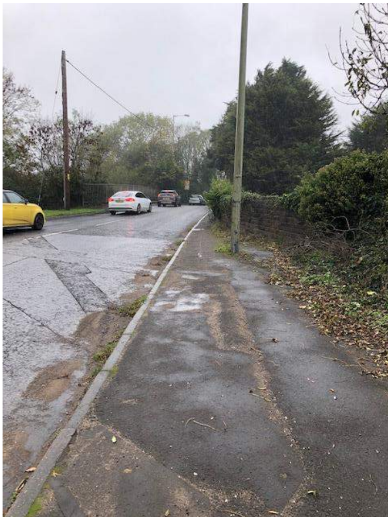
Image 16 – Footways on eastern side of A48 Pyle Road are narrow (Photo: 16/10/18)
