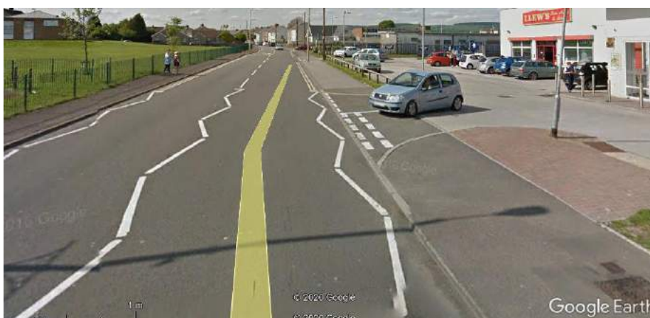
Image 8 – Missing tactile paving Pyle Road (© Google Streetview 05/2016)
