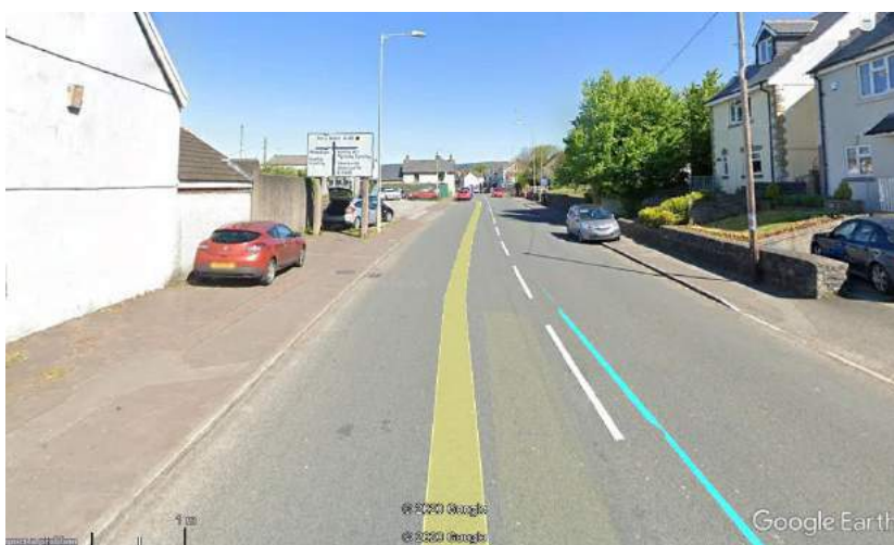
Image 22 – Evidence of on-street parking obstructions on both sides of A48 Pyle Road (© Google Streetview 05/18)
