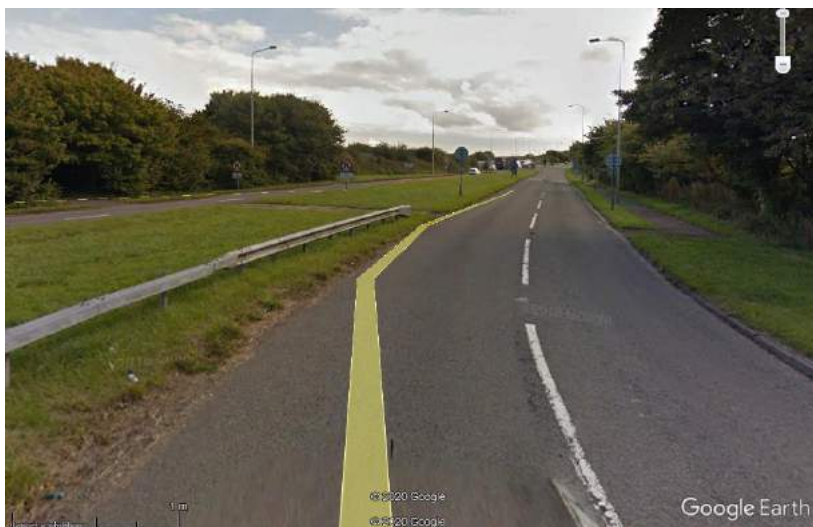
Image 13 – Uncontrolled crossing on A48 north of site near roundabout lacks tactile paving (© Google Streetview 09/15)
