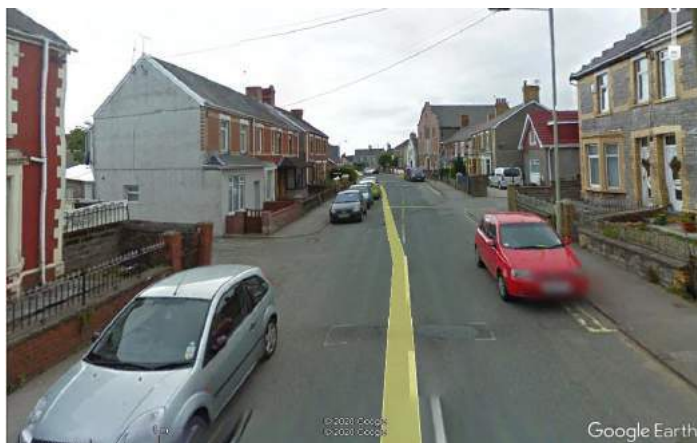
Image 28 – Missing tactile paving and dropped kerb crossing at several junctions along Waun Bant Road. (© Google Streetview 06/11)
