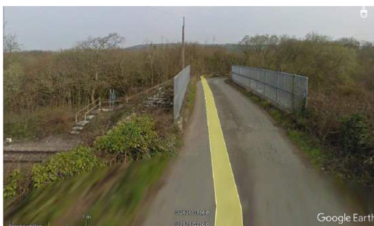
Image 24 – No pedestrian footway over railway bridge leading to Waun Bant Road. Also, no street lighting. (© Google Streetview 03/11)
