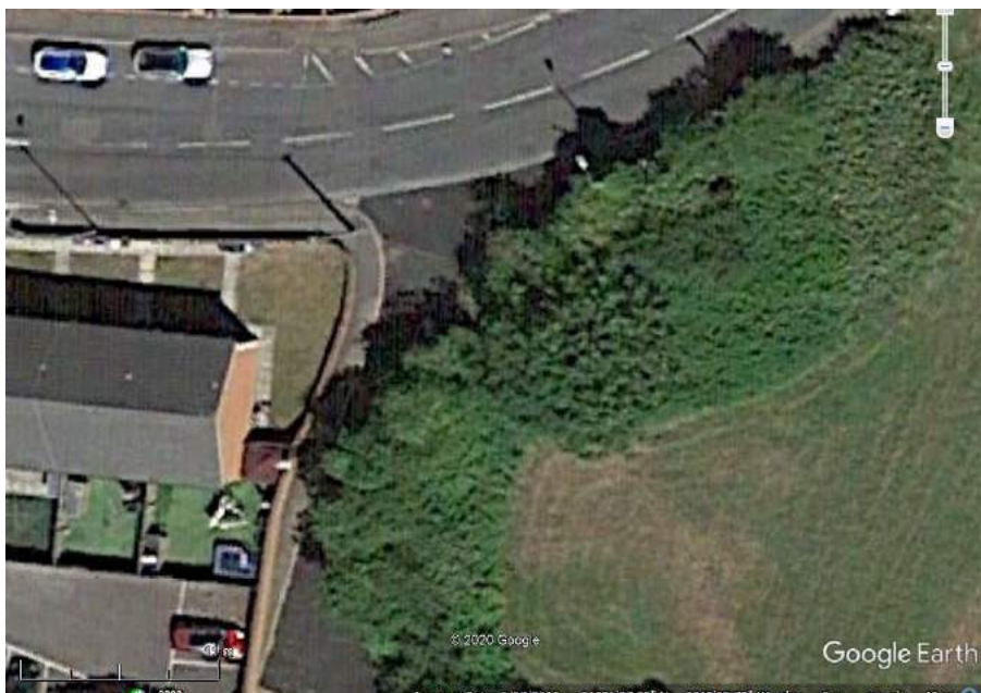
Image 4 – Missing dropped kerbs and tactile paving on Heol Y Sheet junction (© Google Satellite 6/27/2018)
