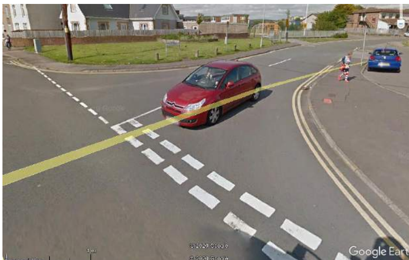
Image 9 – Missing tactile paving on Hall Drive (© Google Streetview 05/2016)
