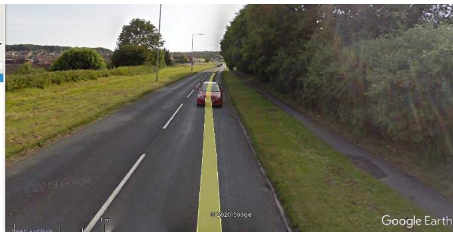
Image 3 – Substandard footway and overgrown foliage on School Terrace but note that suitable footway provision has since been installed on southern side (© Google Streetview 06/11)
