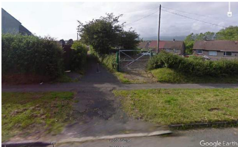
Image 11 – Pedestrian footpath through to Tydraw Crescent is overgrown and lacks lighting (© Google Streetview 06/2011)
