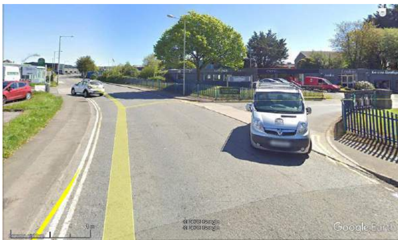
Image 19 – Lack of dropped kerbs and tactile paving at junctions along Heol Mostyn (© Google Streetview 05/18)
