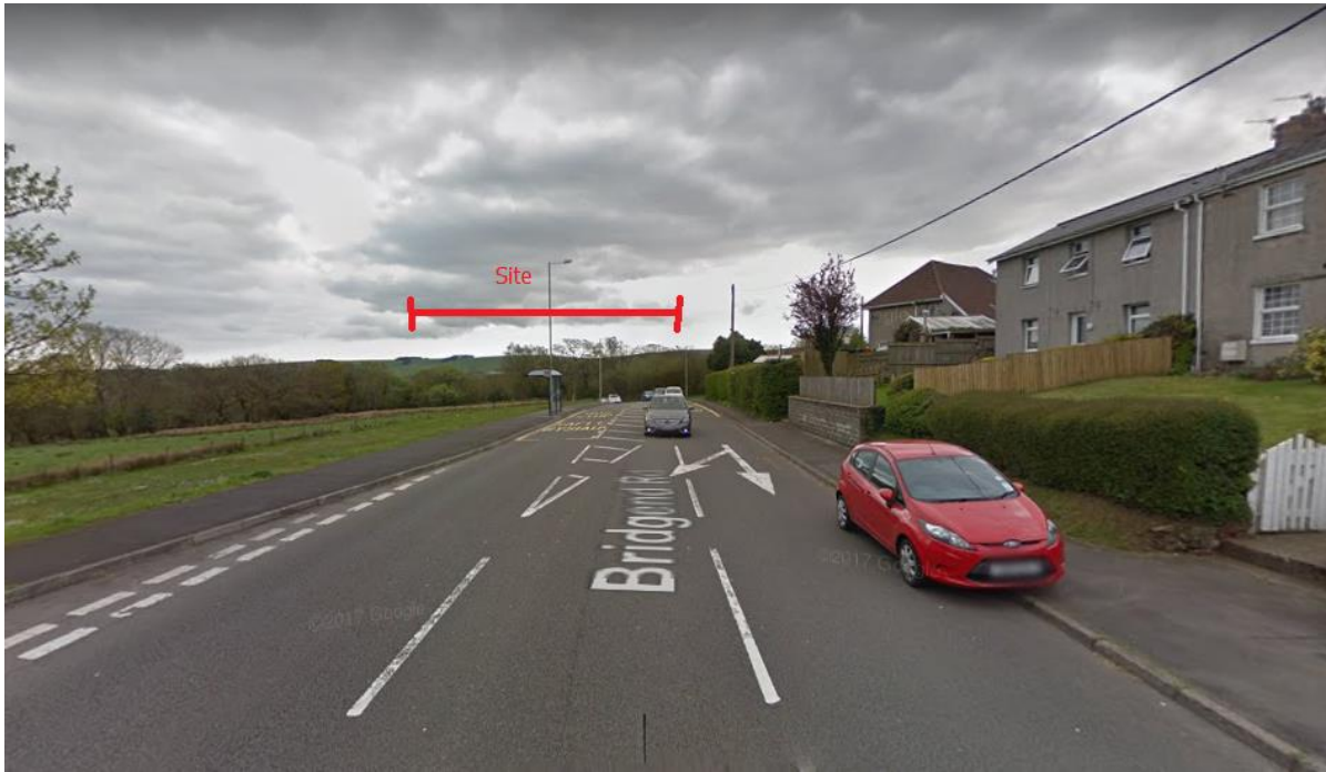
View from North from Bridgend Road
