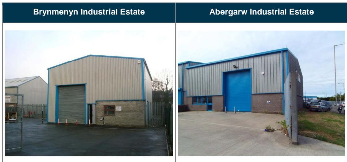
Figure 5.5 Industrial space – Valleys Gateway
