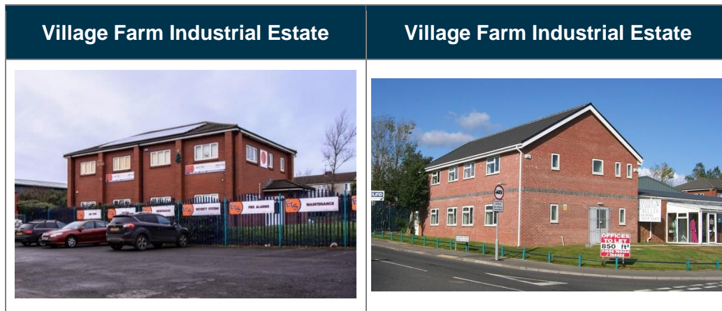
Figure 5.20 Office space - Pyle
